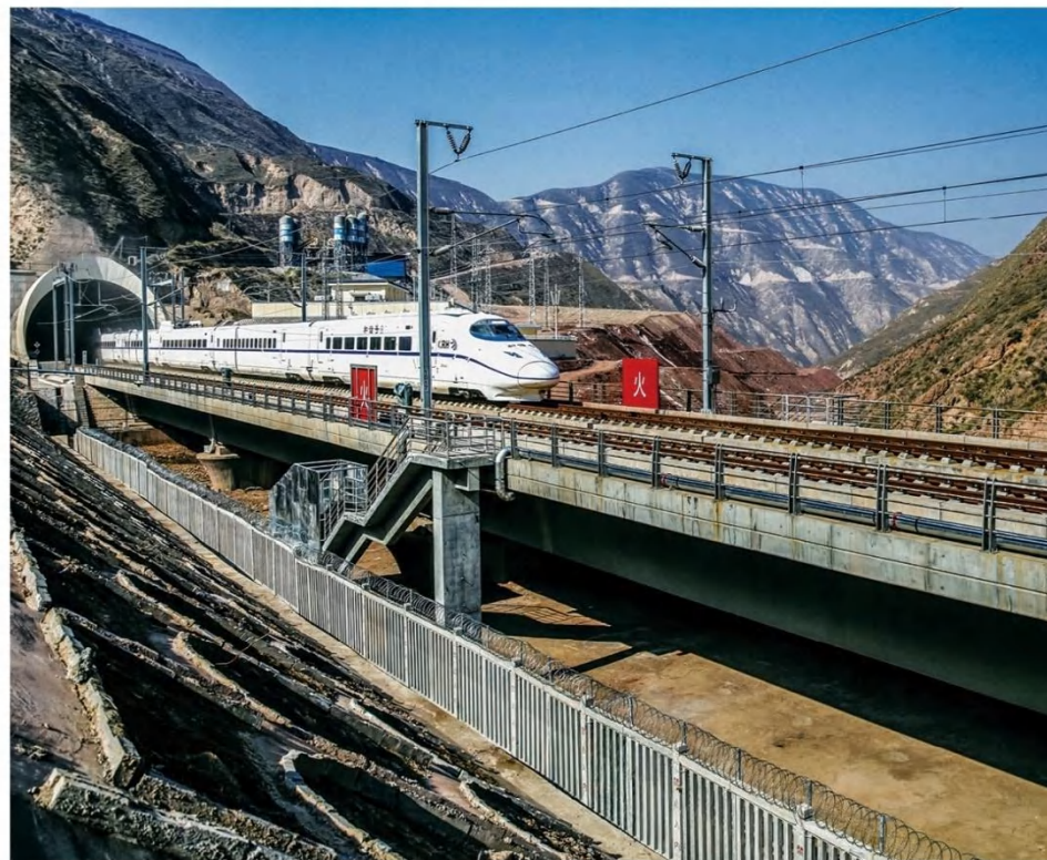
兰(州)新(疆)铁路第二双线 No.2 Double-track of Lanzhou-Xinjiang Railway
