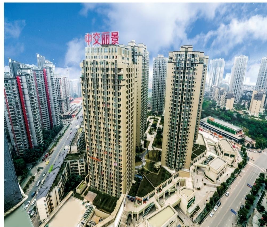
重庆中交丽景七号地块三标段工程 Lot 3 Project of Chongqing CCCC Lijing No. 7 Plot
