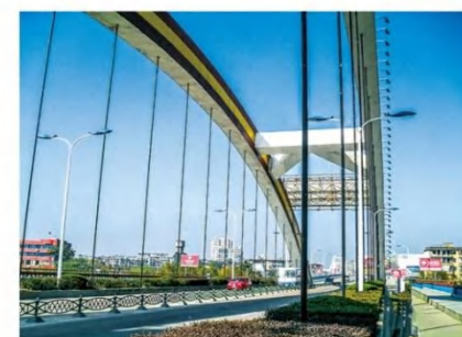
浙江金华市双龙大桥 Shuanglong Bridge in Jinhua, Zhejiang
